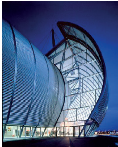
Figura 16. Concert Hall and Exhibition Complex , Bernard Tschumi Architects, Rouen, 2001
